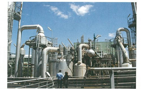
Formaldehyde & resin plant constructed by Chimar
