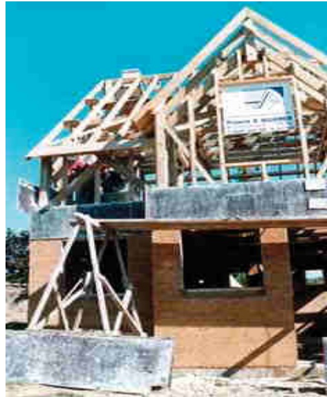
Building in France being constructed entirely of hemp.
